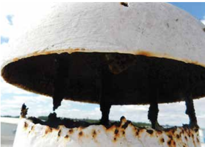
Pittsburg Tank Vent needs replacing because it's allowing rain and wind borne contaminants inside the tank
