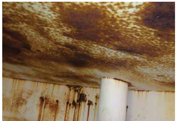
Pittsburg Tank Rust forming on interior roof
