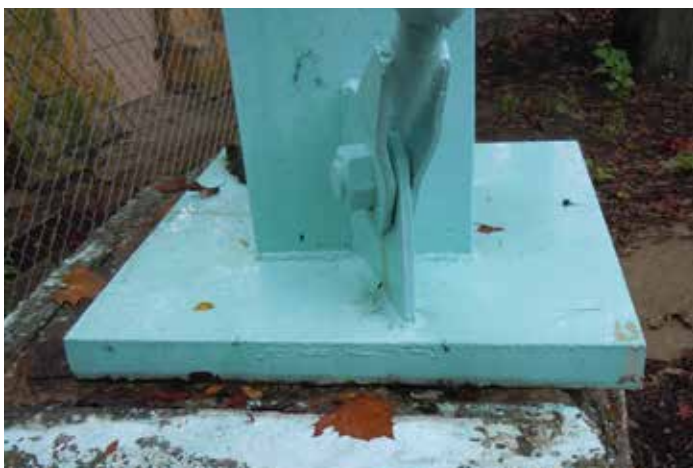
Pittsburg Tank Foundation pier slid off
