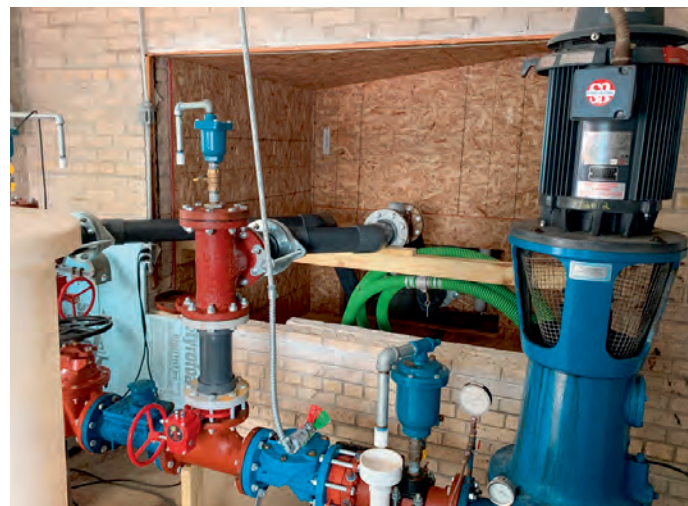
Piping inside the wellhouse, through the temporary connecting structure into the mobile treatment trailer.
