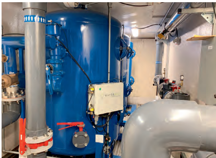
GAC treatment vessels inside the mobile treatment trailer.
