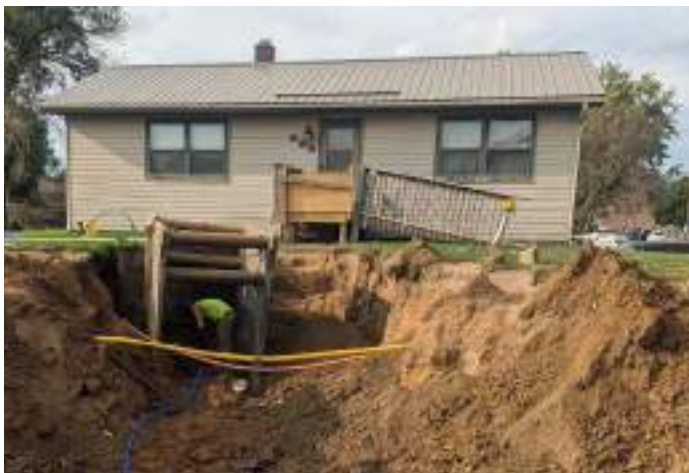
Replacement of water service line
